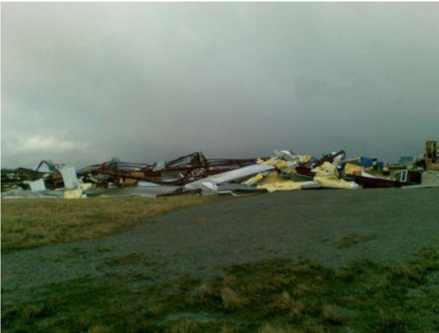
Photo 2: Demolished factory in Greenville, KY
